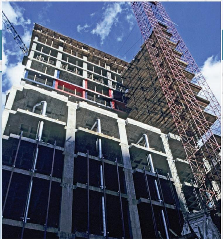
**Laborers also use special supports such as manlifts, personnel hoists and other motorized or movable systems to reach elevated job sites. Each type has its own purposes and characteristics, and each also has specific safety precautions to prevent accidents and injuries.**
